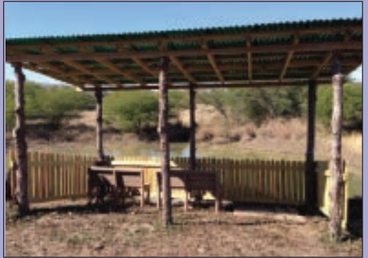
First covered blind at WWBS, by LMN, fencing by Texas State University Students.
