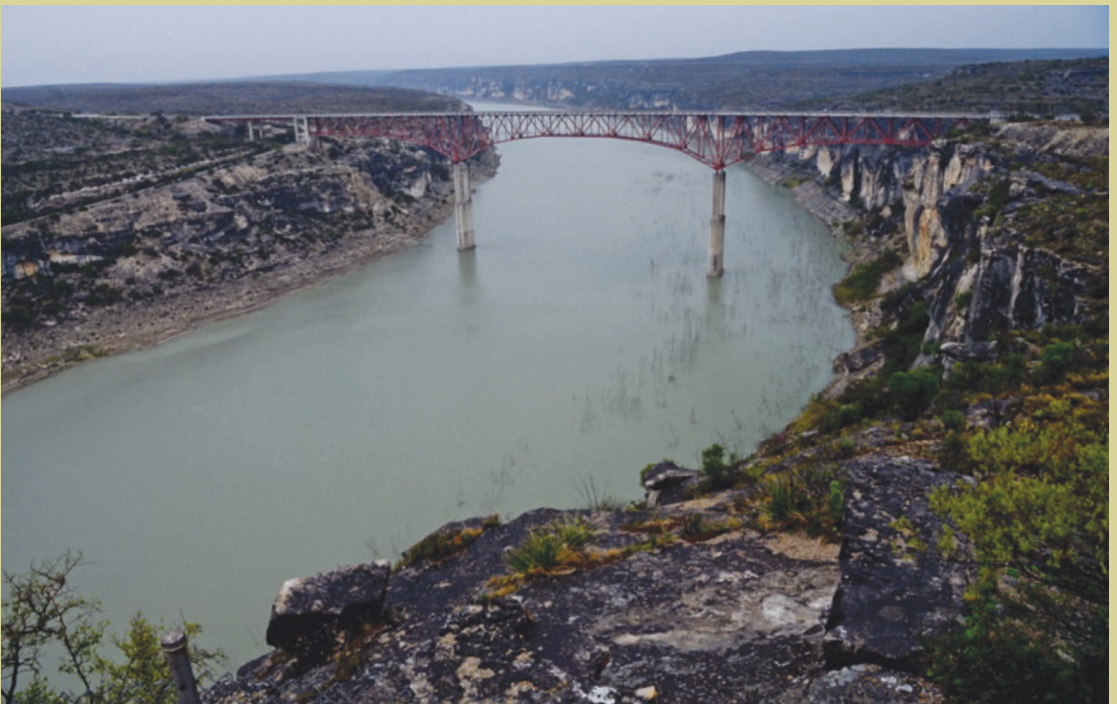
Pecos High Bridge. Despite the rain, I had to stop to take a few bad pictures of this amazing place. This bridge spans 2,180 feet, 321 feet above the river.
