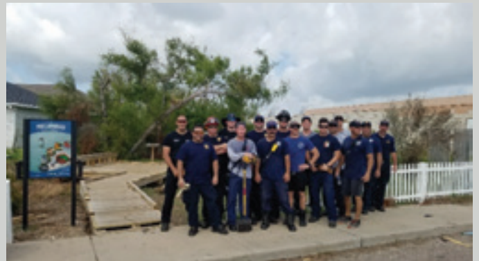
Figure 7. Firefighters helped level the boardwalk by spraying water around each deck piling until it sank back into place. Photo courtesy of City of Port Aransas.
