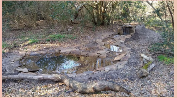
After another load of rocks and just the right arrangement, the pond is finished and ready for the birds and birders on March 19, 2022! Photo credit: James Giroux
