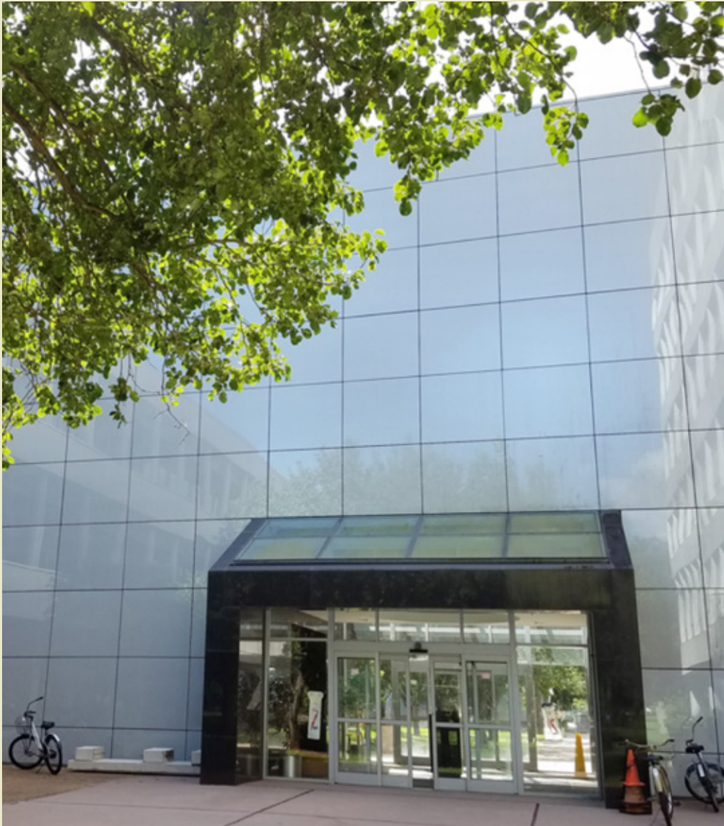
Johnson Space Center's Building 45. Photo by Sandy Parker
