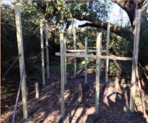
Major supports in place with concrete drying. Photo credit: Dave Dolan
