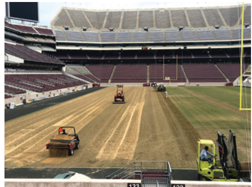
Sodding Kyle Field © Sod Solutions
